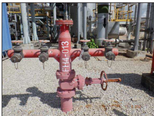
Fire Hydrant/Monitor
